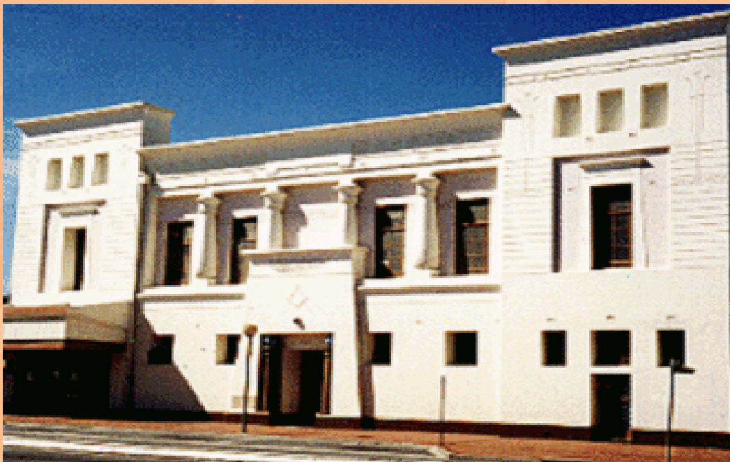
The front of the Masonic Centre at Port Adelaide, South Australia
